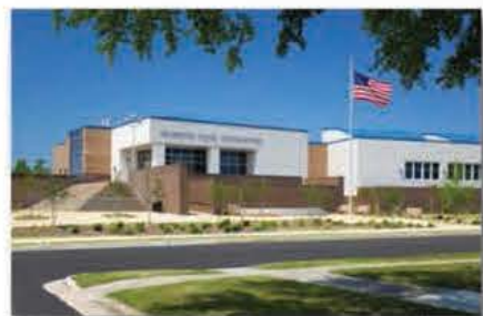
Wilmington Police Headquarters Wilmington, NC
